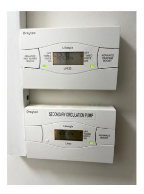
On the upper control panel, press ONCE the right hand button marked ADVANCE HEATING BOOST. This will turn on the heating until it is programmed to next turn off. Pressing the button will cause a green light to illuminate.
